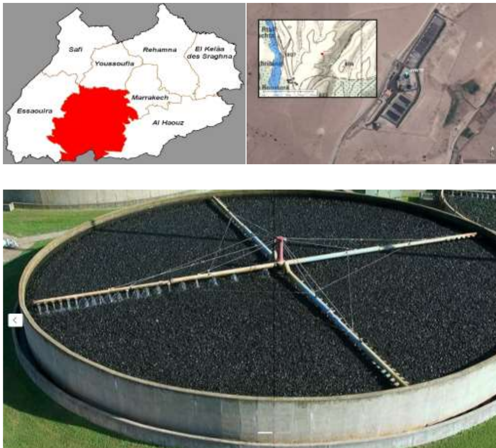
Fig.1. Presentation of the full-scale Bacterial Bed system at Imintanout city (Morocco)
